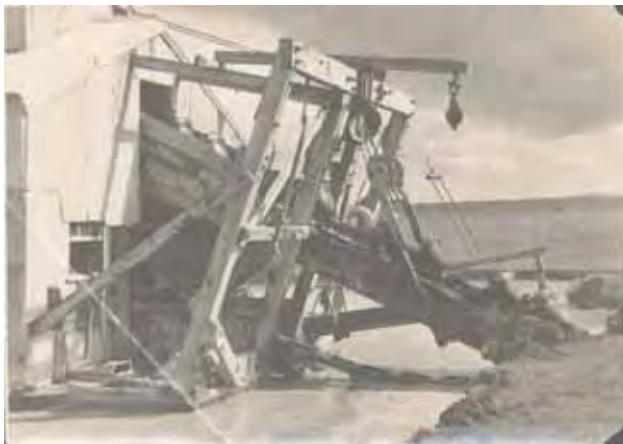
Fig 3 Close-up of buckets stripping topsoil, Waikaka Field. photo Paul Wolperis and Gore District Geological
