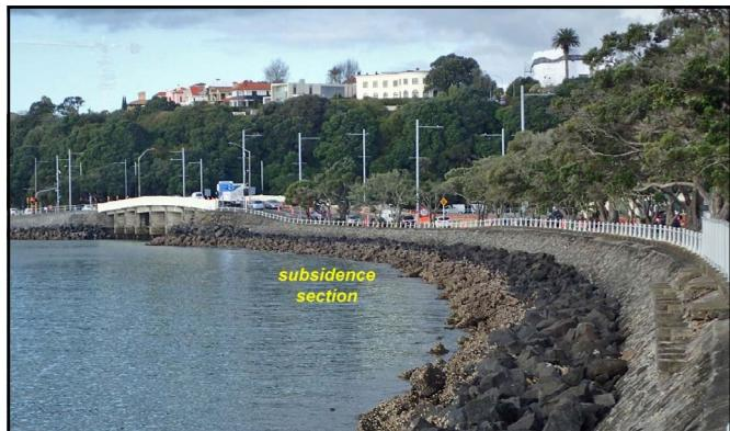
Fig. 1. View east along the outside of Tamaki Drive causeway showing the subsided section above the buried Purewa Stream valley, west of the bridge. Photo: July 2020.
