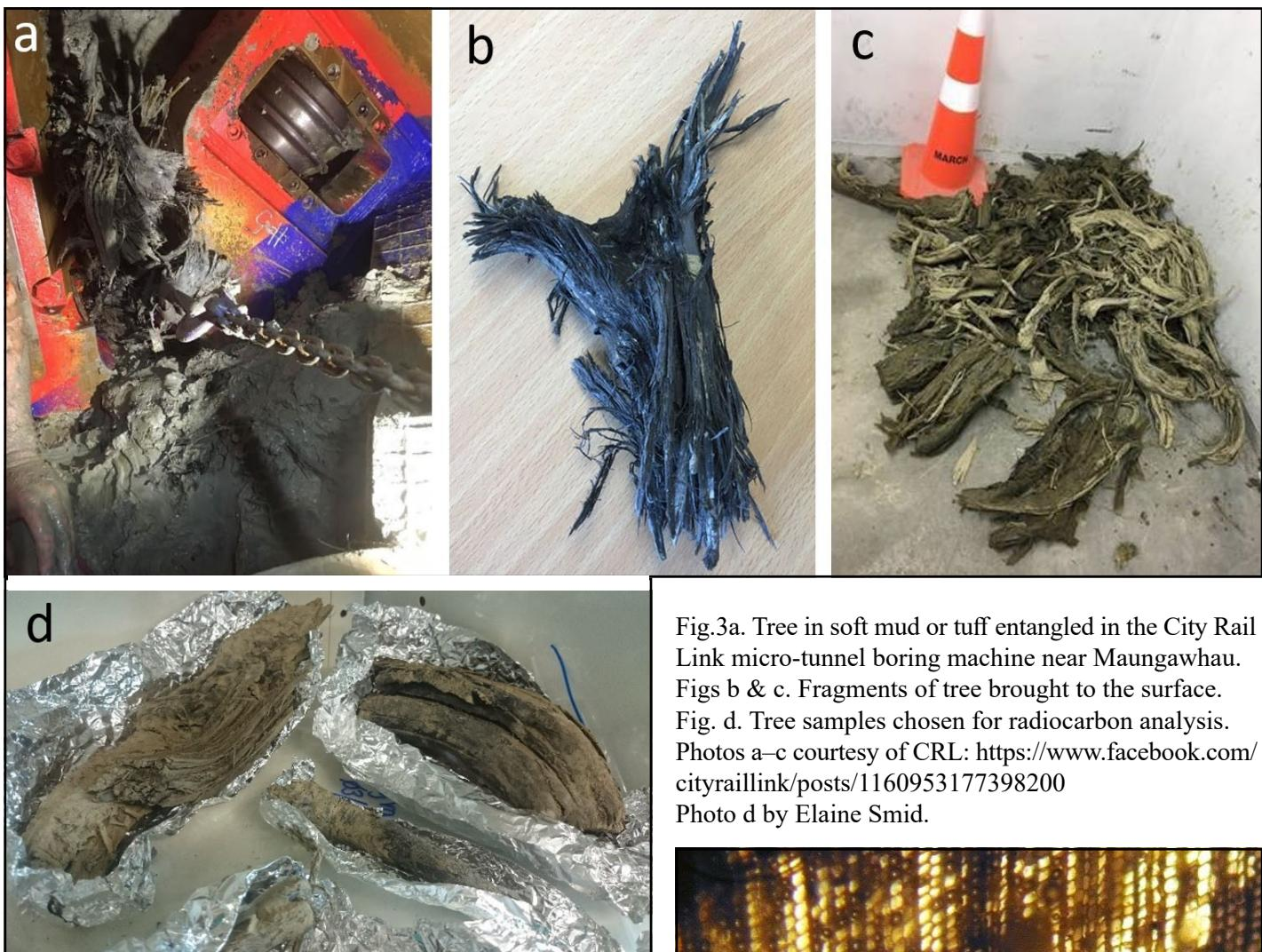
Fig. 3a. Tree in soft mud or tuff entangled in the City Rail Link micro-tunnel boring machine near Maungawhau. Figs b & c. Fragments of tree brought to the surface. Fig. d. Tree samples chosen for radiocarbon analysis. Photos a–c courtesy of CRL: <https://www.facebook.com/cityraillink/posts/1160953177398200>
