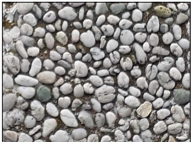
Fig. 5. Exposed aggregate pavement of rounded quartz and occasional argillite pebbles, Kohimaramara.
